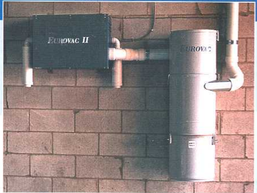
5 HP Eurovac II 2-Man System with Manual Compressed Air PulseJet Cleaning
